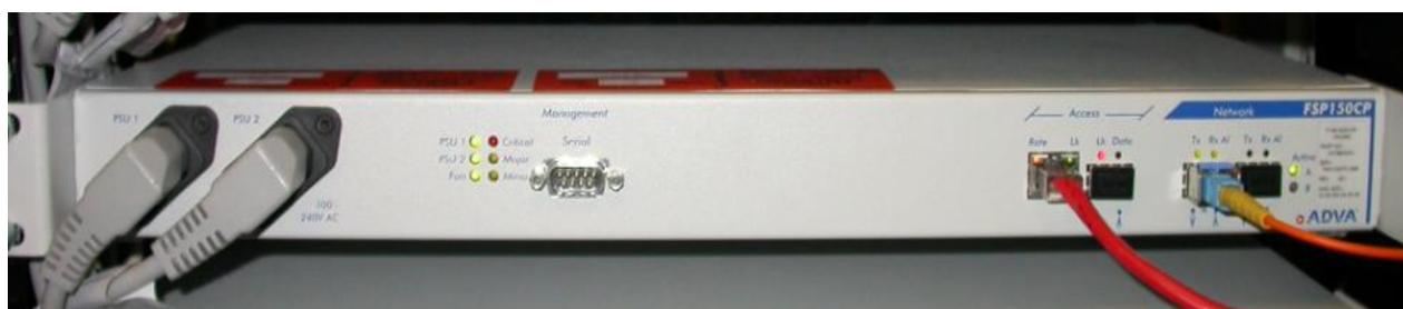
This is what EAD NTE/socket looks like - it is a long white box with a few different sockets for different things. On the left we've got two power supply units plugged in. The "Access" ports are where the EU connects their CPE/equipment and the "Network" port is where BT's fibre comes into the building.
